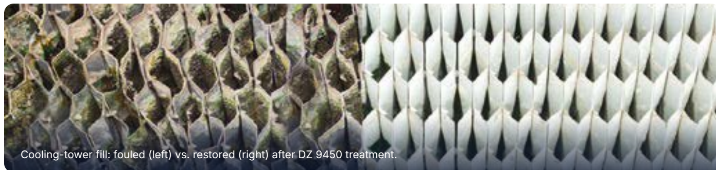
UNDER-DEPOSIT CORROSION IS HALTED ONCE BIOFILM IS REMOVED.
